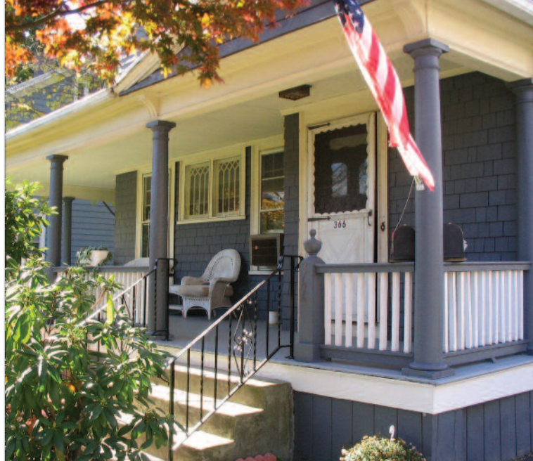
The front porch at Union Avenue
